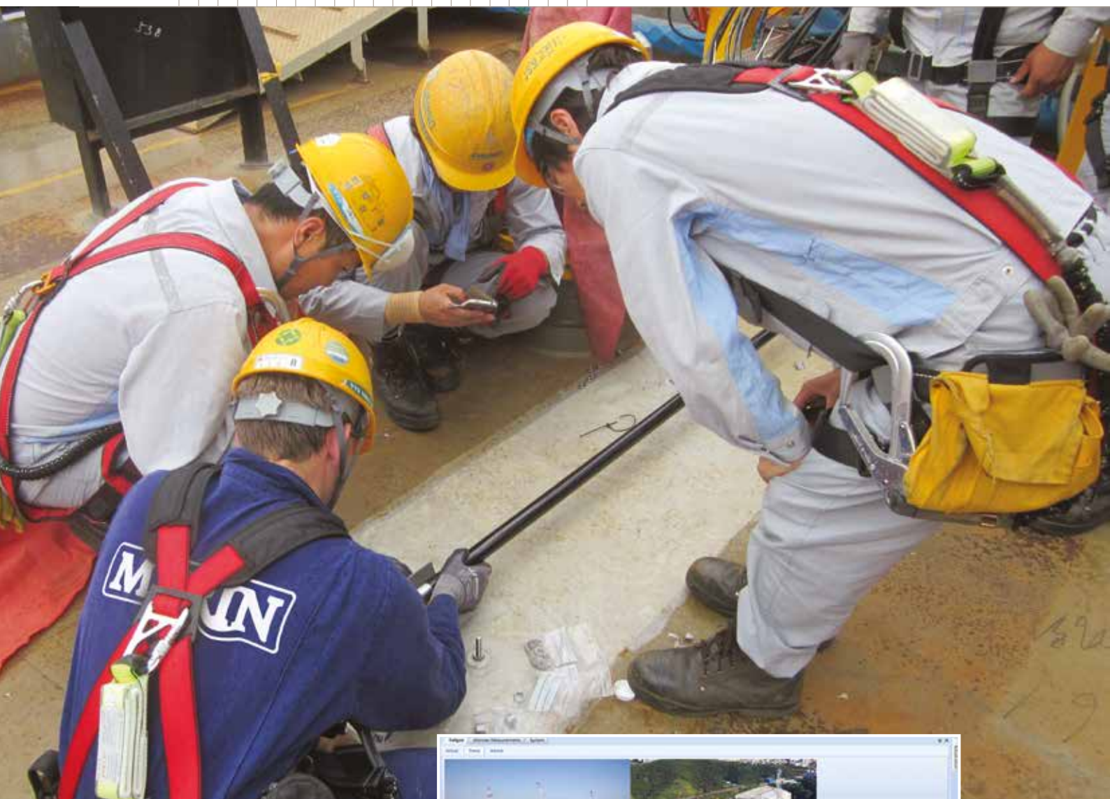
Sensor installation on deck CLOV FPSO
